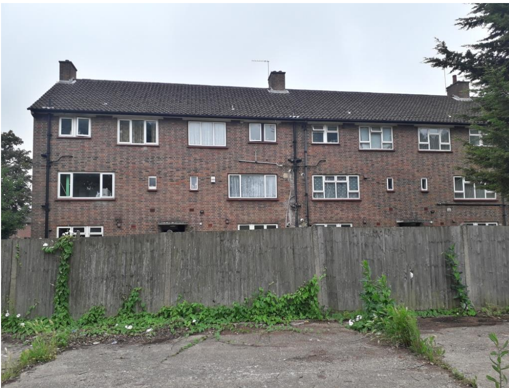
Rear elevation of 386 – 402 Kenton Lane
