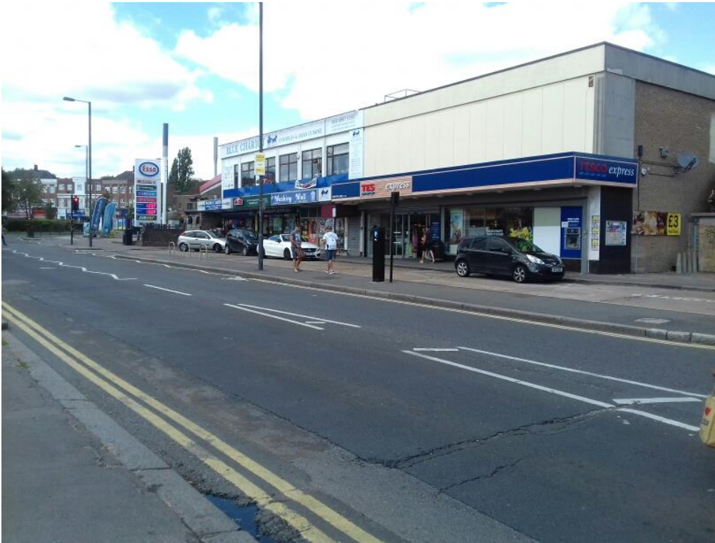
Front elevation of existing Tesco Express
